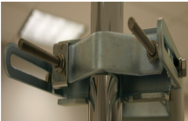
Figure 111 : Attaching the AP antenna upper bracket to the pole
