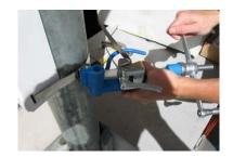
Using the built in cutting tool on the Band-It tool, cut the excess strap.
