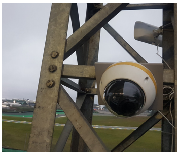
1080p resolution Dahua cameras were used to monitor the area and were connected to the Client MINIs.
