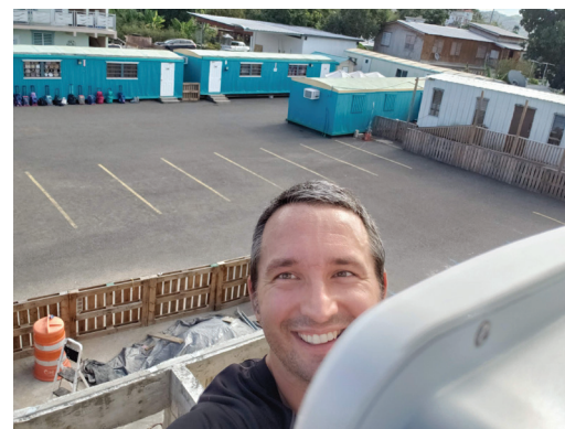
Charlie Galik installs a cnPilot™ e700
