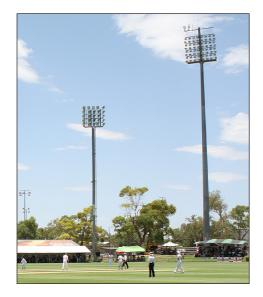
**Wireless Access** - Solutions were mounted to the top of the lighting towers to provide near Alice-wide backhaul connectivity and connected into the PTP500 backhaul. Because of their location in the stadium, additional access network subscriber modules can be installed to extend coverage into the surrounding area as needed in the future.
