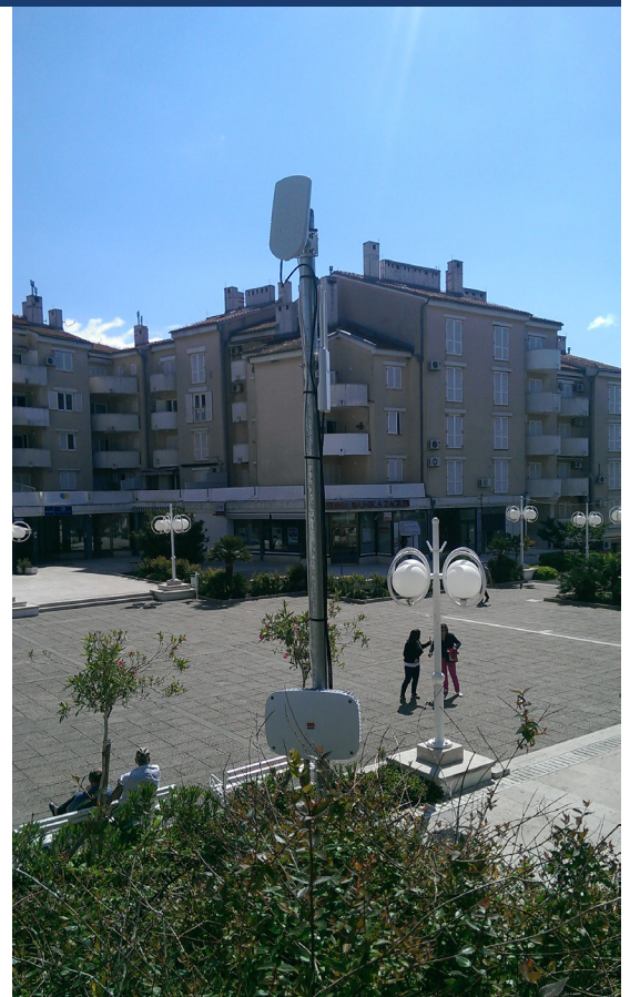
ePMP Subscriber Module connects a Public WiFi Access Point
